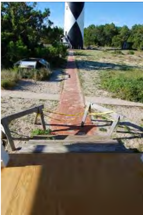
FIGURE 103. Brick walk at the front of the Keeper's Dwelling leading to the lighthouse, with the perpendicular concrete path also visible.
