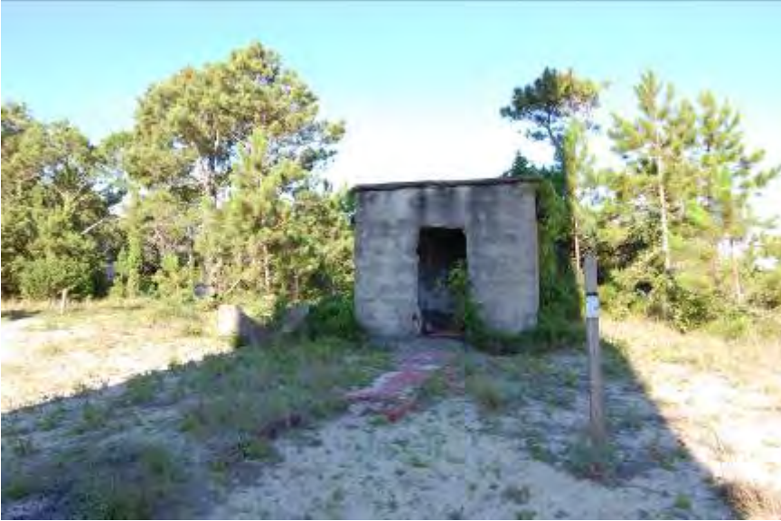
FIGURE 45. The cast-in-place concrete oil house is located west of the lighthouse.
