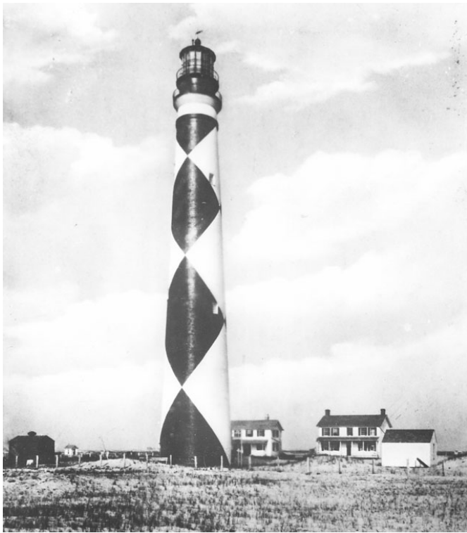
FIGURE 41. Lighthouse Complex, looking west, circa 1913. Copy of hand-colored post card from Beaufort Drug Company.
