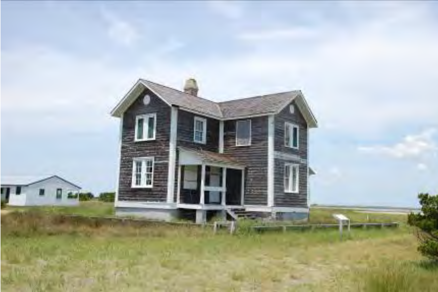
FIGURE 61. Similar view to Figure 60 , the rear kitchen porch of the Barden House. The Barden House has been located near the shore of the bight on a concrete block foundation since 1958.
