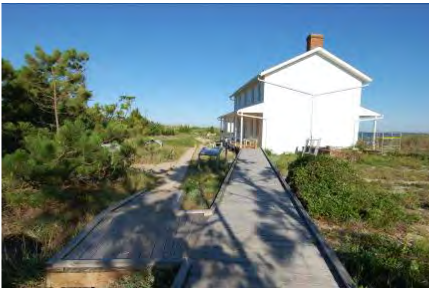
FIGURE 104. The eastern extent of the concrete walkway adjoins the raised wooden boardwalk that accesses the Keeper's Dwelling to the west and also continues east towards the lighthouse dock.
