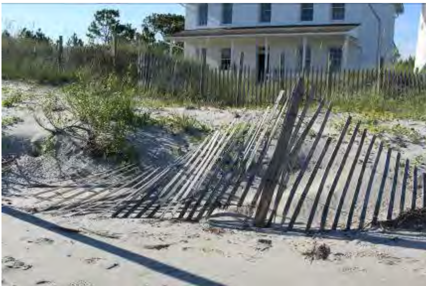
FIGURE 151. Fencing for dune stabilization along the beach adjacent to the Keeper's Dwelling.
