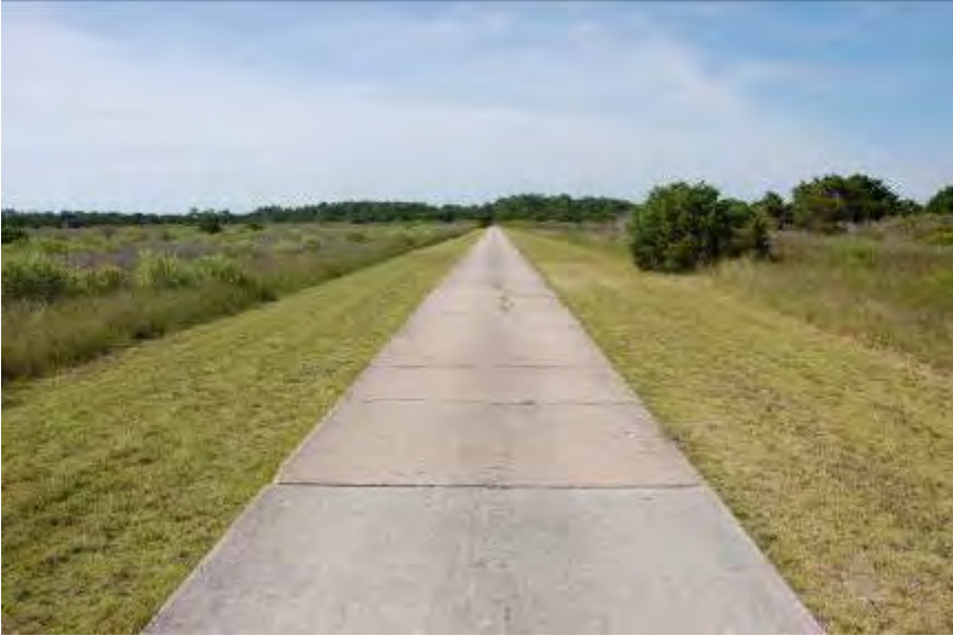
FIGURE 113. The Concrete Road leads between the former Coast Guard Station and the Coast Guard dock.
