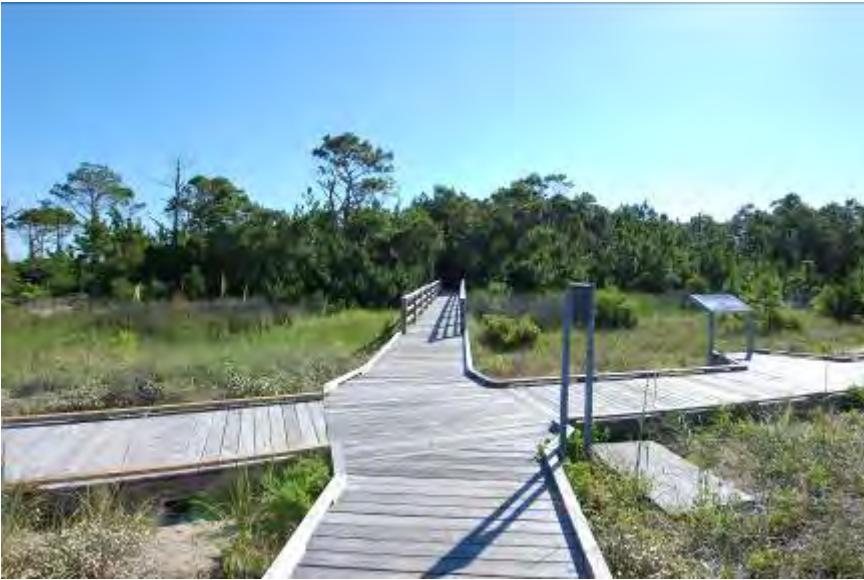
FIGURE 106. Raised wooden boardwalk that connects sections of the Lighthouse Complex.
