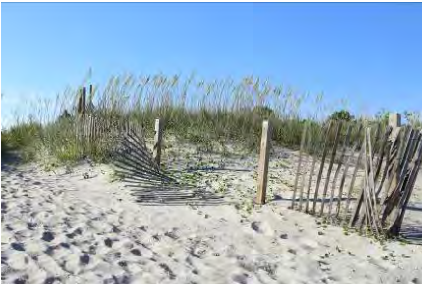
FIGURE 150. Fencing for dune stabilization along the beach adjacent to the Keeper's Dwelling.
