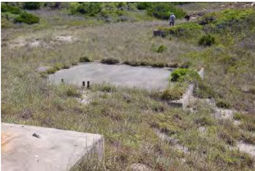
FIGURE 181. Concrete foundations associated with World War II-era military activity.
