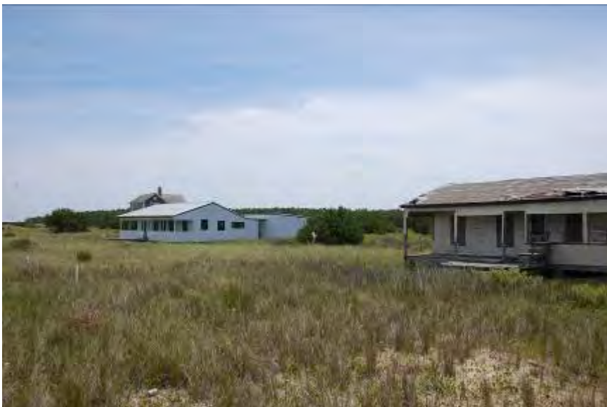
FIGURE 184. The Jetty Workers House #1 and Jetty Workers House #2 (left and right) with the roof of the Barden House in the background.
