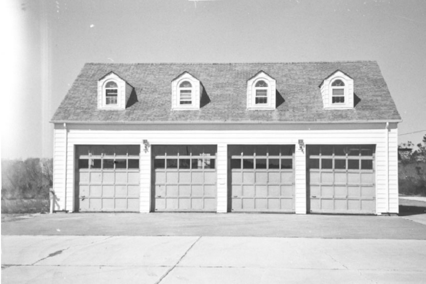
FIGURE 87. Cape Lookout Coast Guard Station garage, looking west, post-1939.
