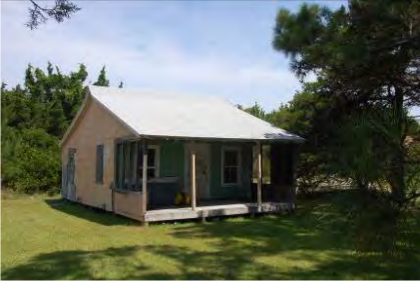
FIGURE 71. The O'Boyle-Bryant House is a one-story wood frame cottage.
