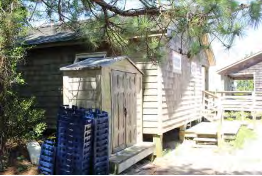
FIGURE 170. Showering platform on side of comfort station building and small NPS shed on back side.
