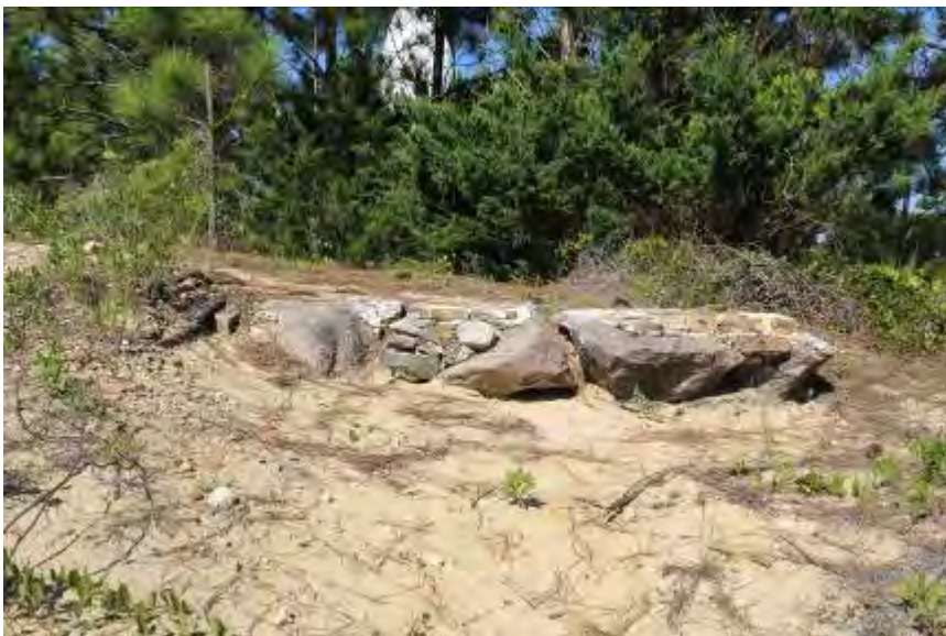
FIGURE 178. Stone and brick rubble foundation remnants.
