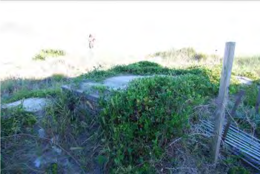
FIGURE 51. The 1907 brick cistern west of the 1907 Keeper's Dwelling.
