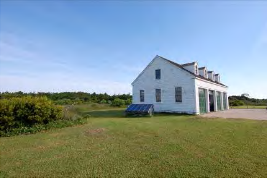
FIGURE 160. The former Coast Guard Station Complex generates power through solar panels located in the yard around the Coast Guard Garage.
