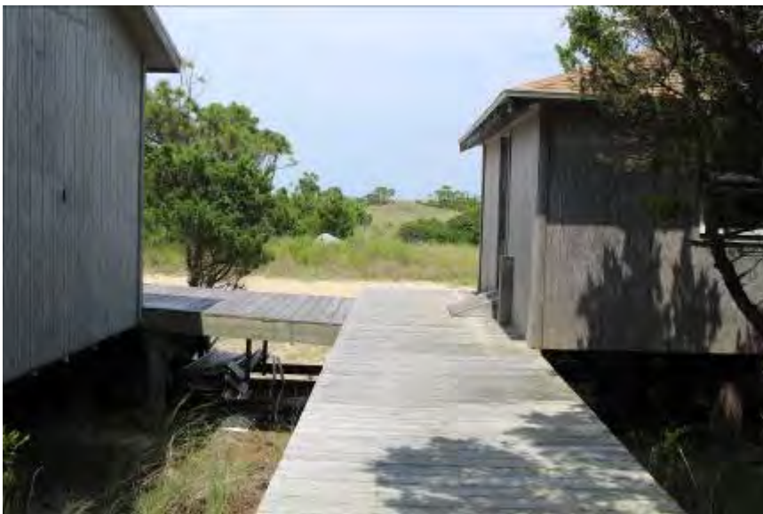
FIGURE 109. Raised boardwalk at Les and Sally Moore Complex that accesses the NPS outbuildings to the southeast of the main house.
