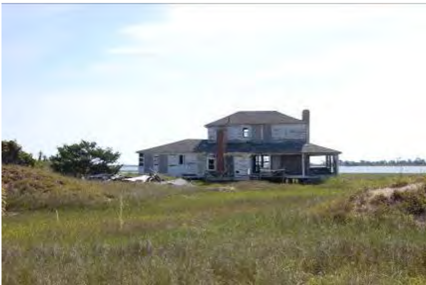
FIGURE 94. The Casablanca House sits near the Coast Guard dock on the northern end of Concrete Road.
