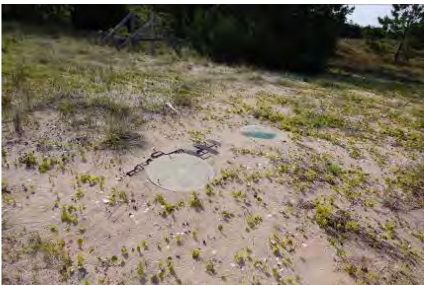
FIGURE 165. Manhole covers are examples of the many water related small-scale features at the Coast Guard Station.
