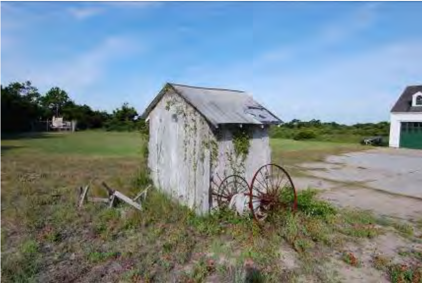
FIGURE 171. A hose reel edges the former Coast Guard Station parking lot.
