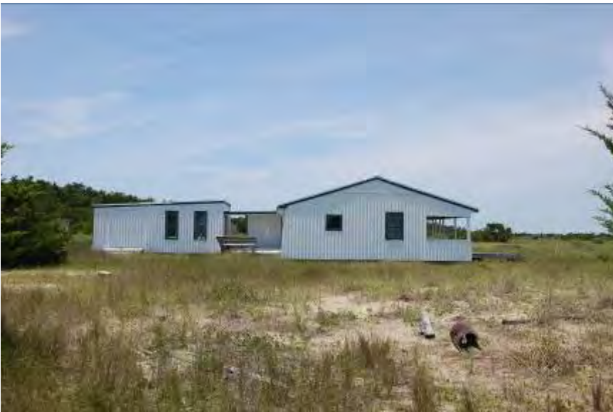
FIGURE 62. Jetty Workers House #1 is connected to its garage via a breezeway and was renovated in circa 2013.
