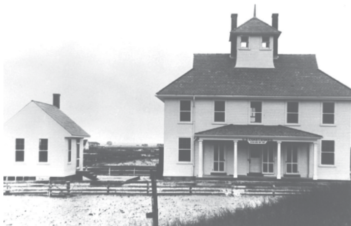
FIGURE 15. The newly-constructed Coast Guard Station and kitchen building, circa 1917. A number of buildings in the Cape Lookout Village can be seen in the distance between the two station buildings (arrows).
