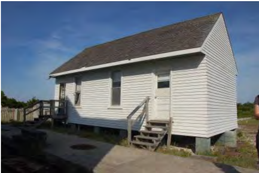
FIGURE 84. The Coast Guard summer kitchen is a one-story building adjacent to the main building, with the summer kitchen cistern foundation in the foreground.
