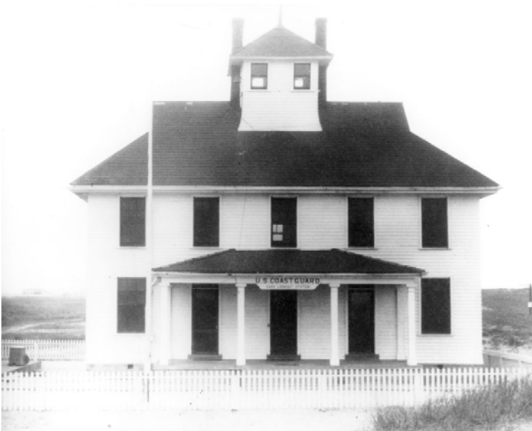
FIGURE 79. Cape Lookout Coast Guard Station main building, looking north, circa 1939.
