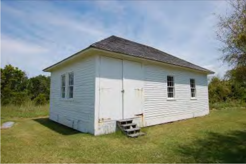
FIGURE 69. The Yeomans House (original Coast Guard Station Boathouse) was rehabilitated in circa 2009.
