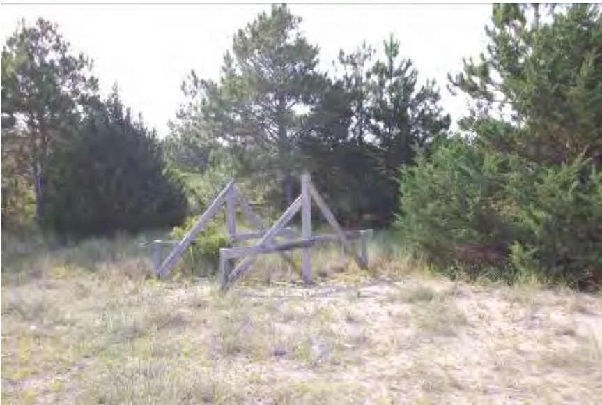
FIGURE 161. Wooden structures at Coast Guard Station that previously supported solar panels.
