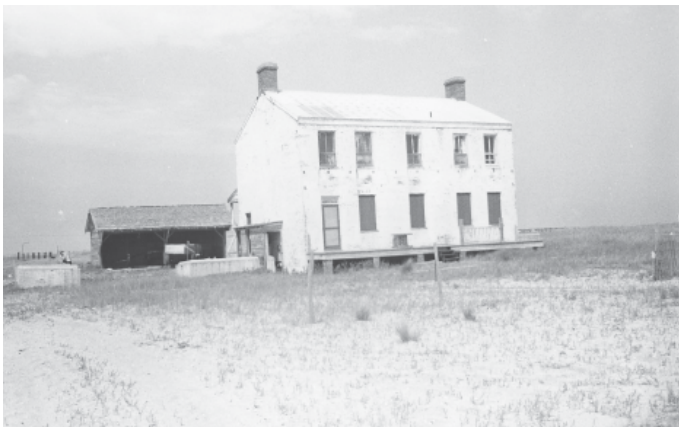
FIGURE 36. 1873 Keeper's Dwelling and coal shed, 1970 condition survey photograph. Note the wooden lean-to at the west gable wall of the dwelling and the absence of a porch across the south side of the building.
