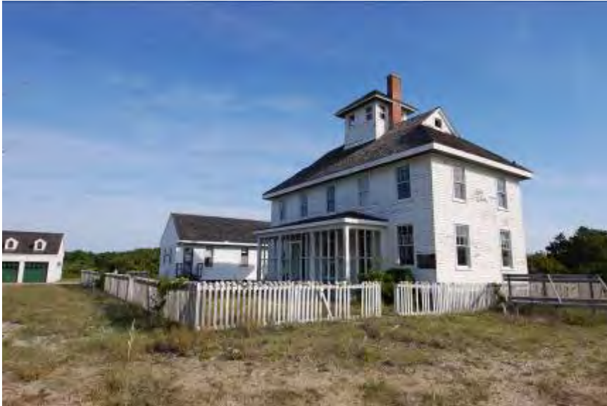
FIGURE 83. The Cape Lookout Coast Guard Station main building was constructed in 1916–1917.
