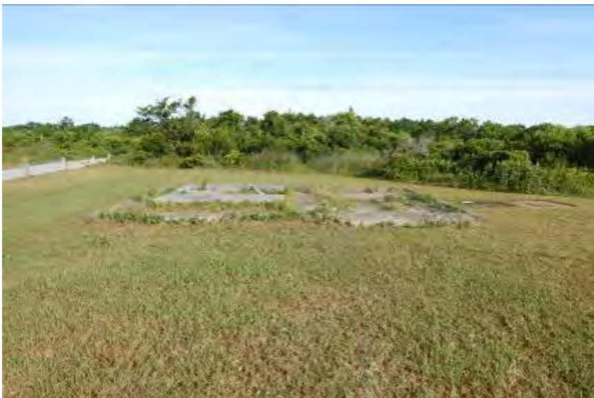
FIGURE 91. This concrete foundation north of the Coast Guard garage marks the location of the former Navy "Power House" incinerator/generator shed.
