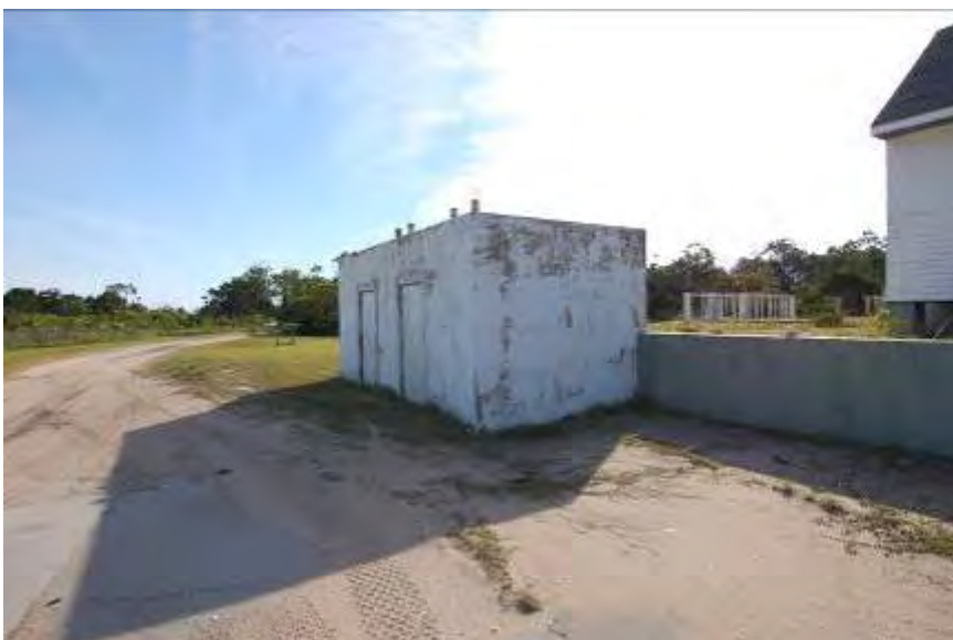
FIGURE 92. Built into the retaining wall at the Coast Guard station is a concrete cistern building.
