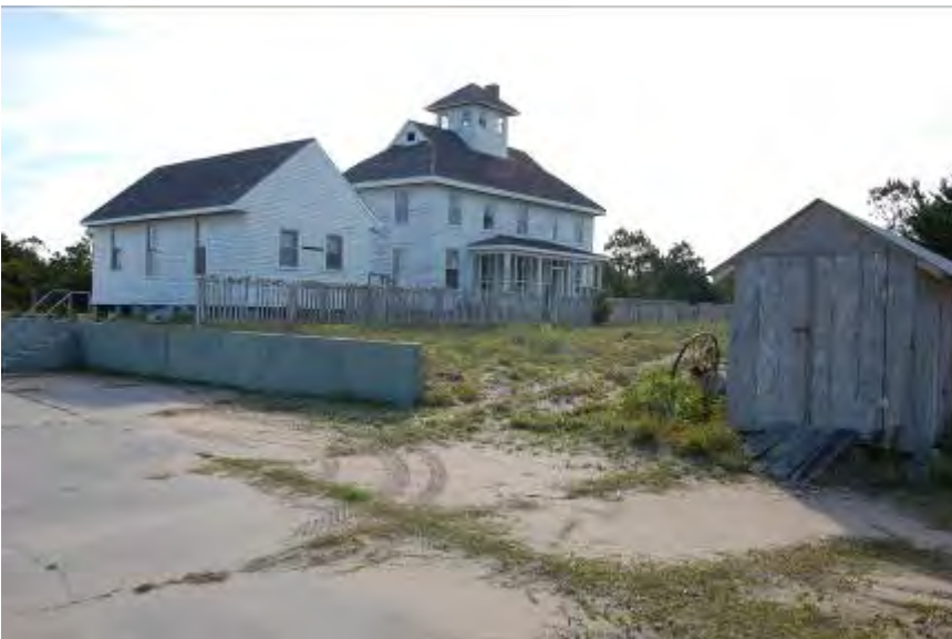
FIGURE 82. The same view as Figure 81 toward the Cape Lookout Coast Guard Station. An electrical pole has been removed from behind the summer kitchen, and conduit removed from the side of the summer kitchen. The antenna has been removed from the top of the cupola over the main building. The wooden shed has been added to the station.
