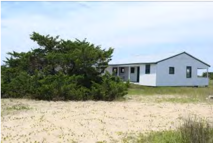
FIGURE 128. An area that has experienced a washover. Note the sand deposits.
