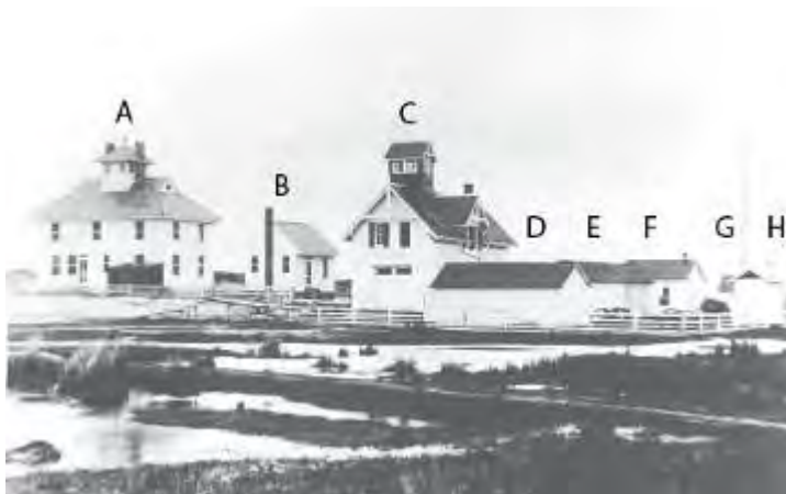
FIGURE 16. The Coast Guard Station circa 1917, looking south. Note the standing water and swampy conditions in the foreground. A: 1917 Coast Guard station main building; B: 1917 kitchen; C: 1887 Life-Saving Station, relocated 1916; D: 1892 boathouse; E: 1892 stable; F: 1892 kitchen, relocated 1917; G: 1888 storage building, relocated 1917; H: privy.
