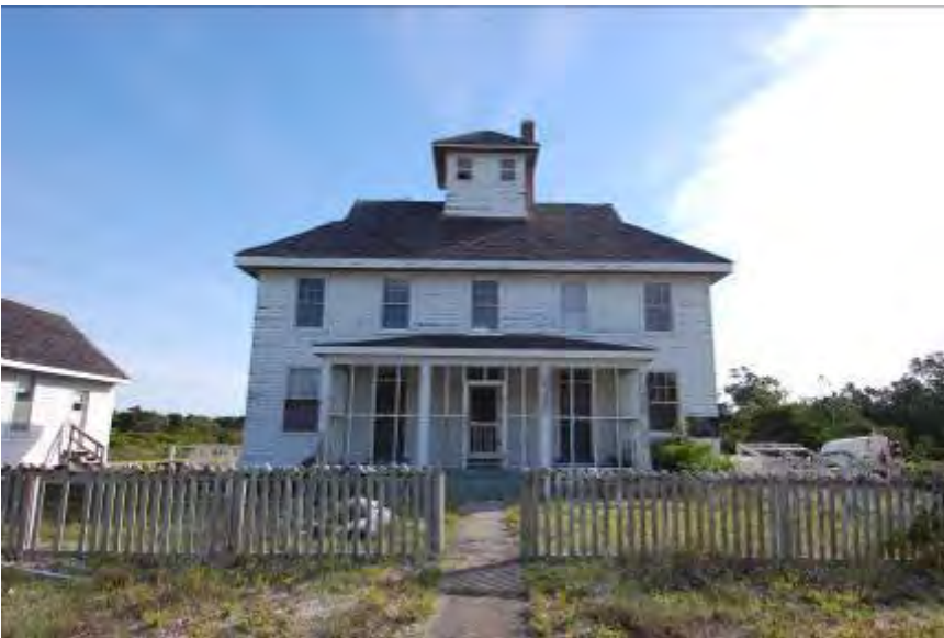
FIGURE 80. The same view as Figure 79 toward the Cape Lookout Coast Guard Station. Note, the sign has been removed and a screened porch added (though no screening was present at time of survey). A gate has been added in the picket fence, and welk shells placed over the tops of the pickets. A chimney has been removed from the left side of the cupola. A wooden structure on which solar panels were previously mounted is visible to the right of the station.
