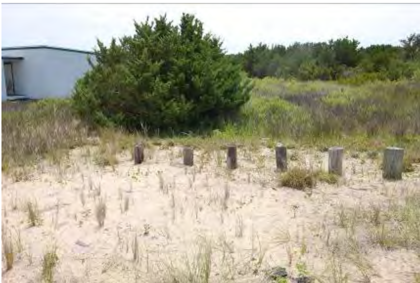
FIGURE 154. Bollard edging composed of treated pilings adjacent to the Jetty Workers House #1.
