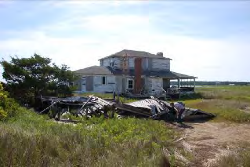
FIGURE 95. Collapsed sheds in front of the Casablanca House.
