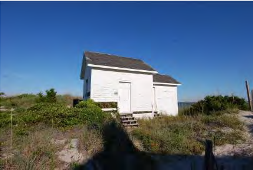
FIGURE 50. The 1907 summer kitchen west of the Keeper's Dwelling near the shoreline.
