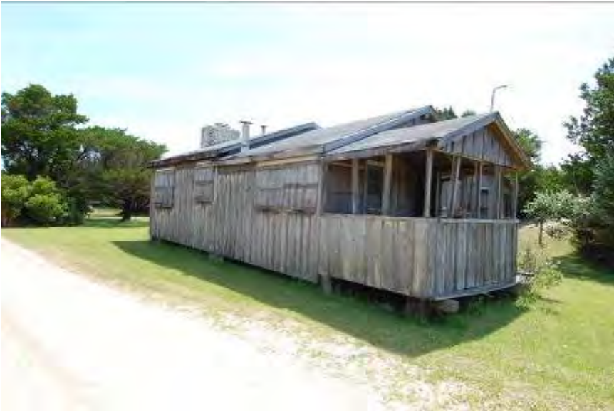
FIGURE 68. The Setzer-Dawsey House is clad in unpainted wood board and batten siding.
