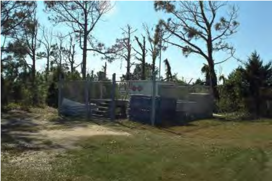
FIGURE 159. Chain link fencing edges utility boxes near the former Coast Guard Station.
