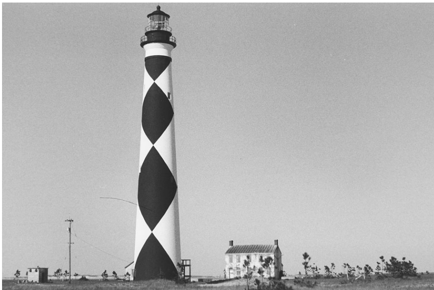
FIGURE 42. Lighthouse Complex, looking west, circa 1979.
