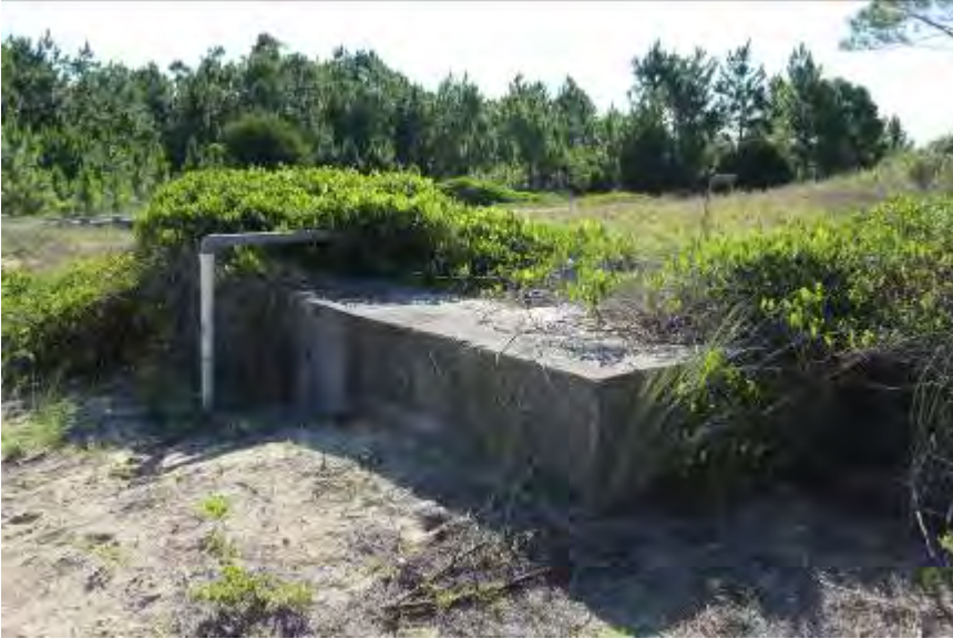
FIGURE 168. Large above ground cistern located to the south of the lighthouse.
