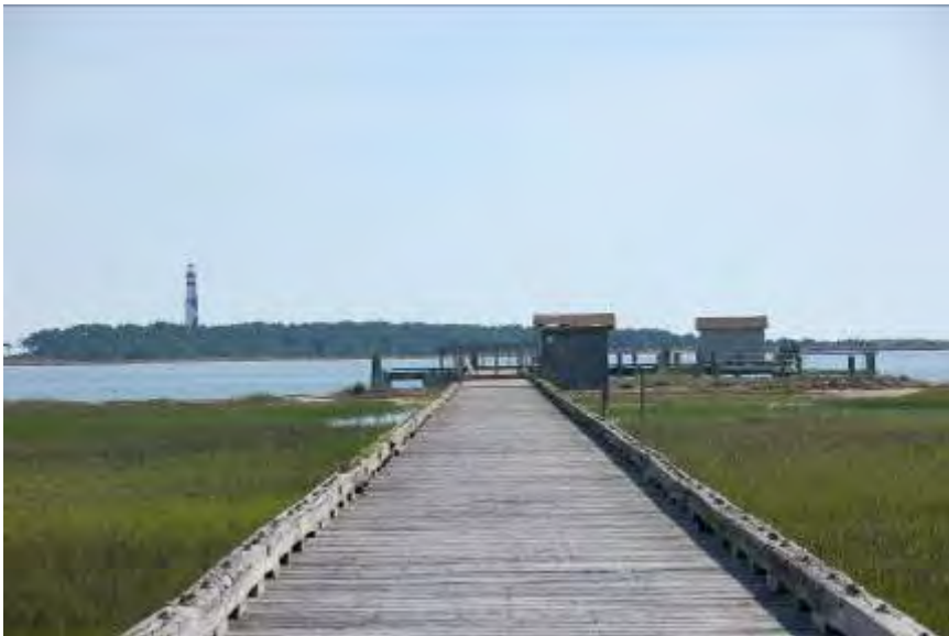
FIGURE 99. Storage sheds on the far side of the Coast Guard dock.
