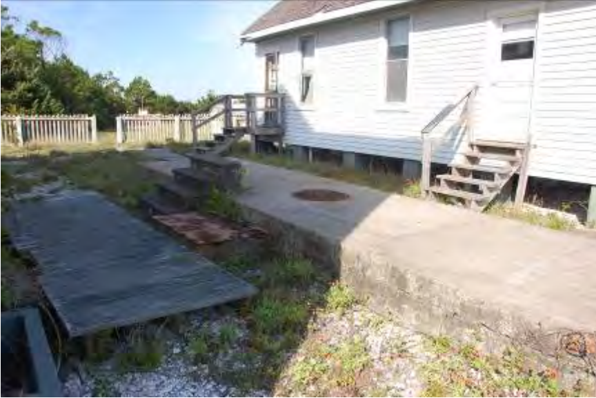
FIGURE 85. The summer kitchen (right) and associated summer kitchen cistern foundation.
