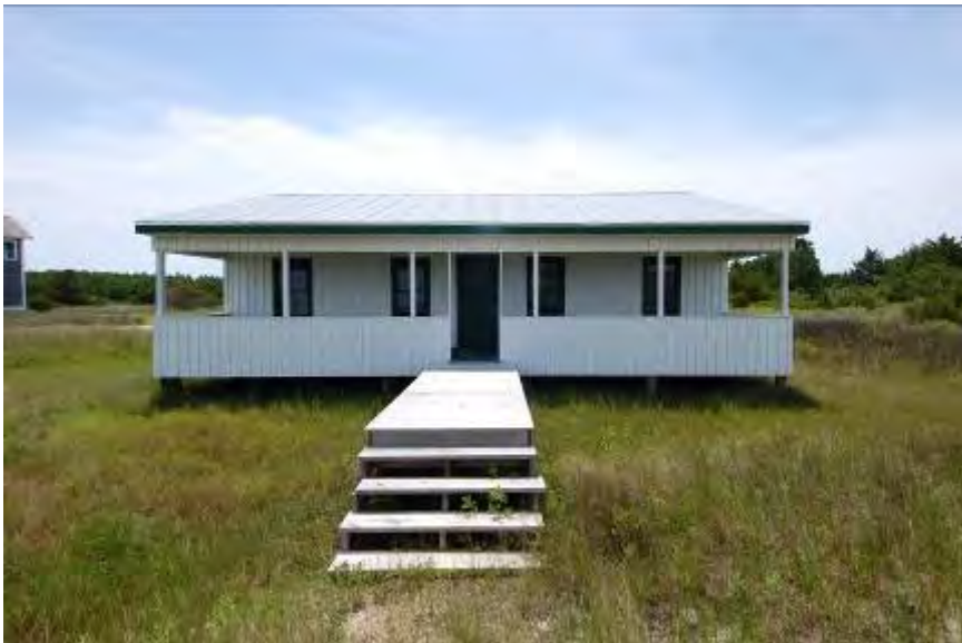
FIGURE 63. Jetty Workers House #1 entry boardwalk.
