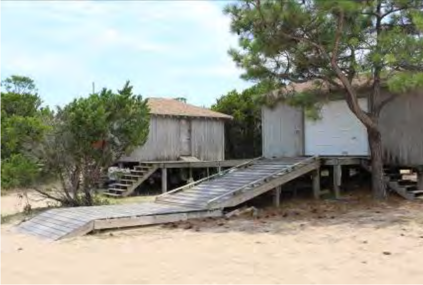
FIGURE 57. Adjacent to the Les and Sally Moore Complex are three NPS buildings: a generator shed (left), a garage (center), and a storage shed (beyond trees at right outside of photo frame).
