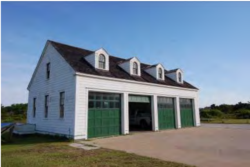
FIGURE 89. The four bay garage at the Coast Guard station. Note the downspouts and carriage lights have been removed.
