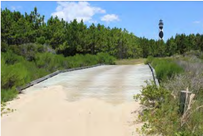
FIGURE 111. An example of a wooden bridge that crosses an intermittent drainageway.
