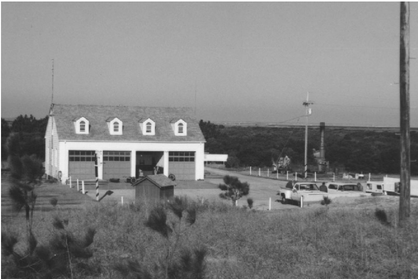
FIGURE 88. Cape Lookout Coast Guard Station garage, looking northwest, circa 1979.
