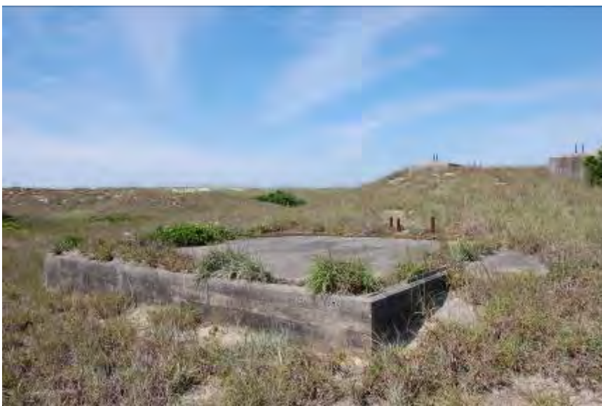
FIGURE 179. Concrete foundations associated with World War II-era military activity.
