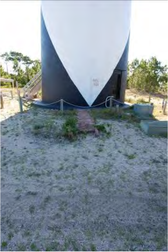
FIGURE 144. Wood posts with rope encircle the lighthouse.
