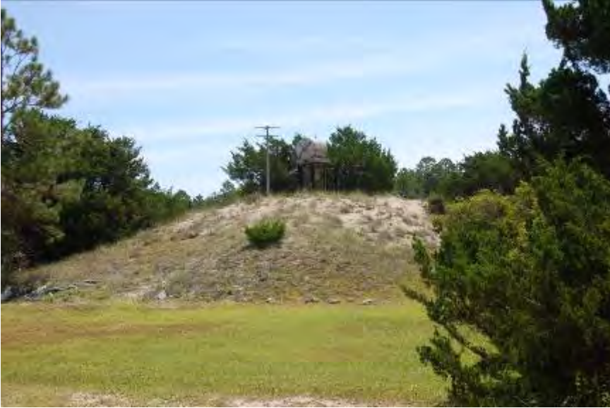
FIGURE 158. Utility pole and raised gas storage tank on hill adjacent to Setzer-Dawsey House.
