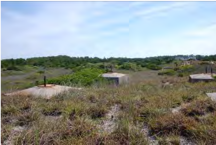
FIGURE 180. Concrete foundations associated with World War II-era military activity.
