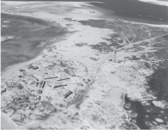
FIGURE 27. Aerial view circa 1940s looking northeast, showing the World War II army camp.
