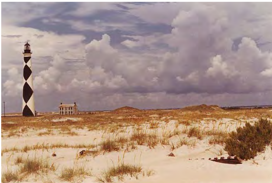
FIGURE 31. Cape Lookout Light Station, view from the southeast, circa 1960s.
